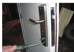
If door handles are packed with tension removed. Remove circlip & tension as detail. Replace circlip.
